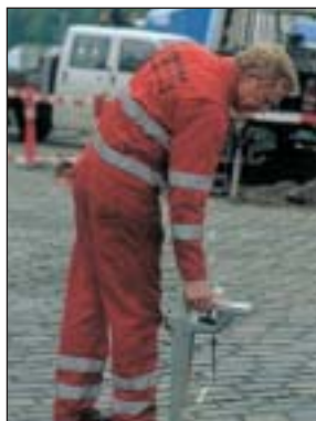
Successful pipe bursting requires thorough preliminary surveying.
