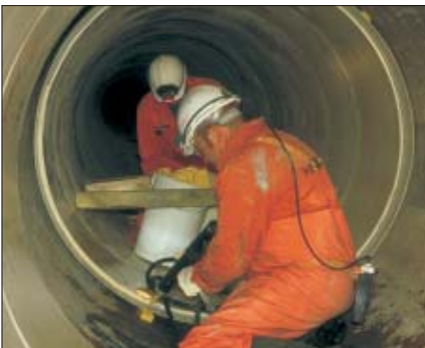
Fastening panels to the existing pipeline.
