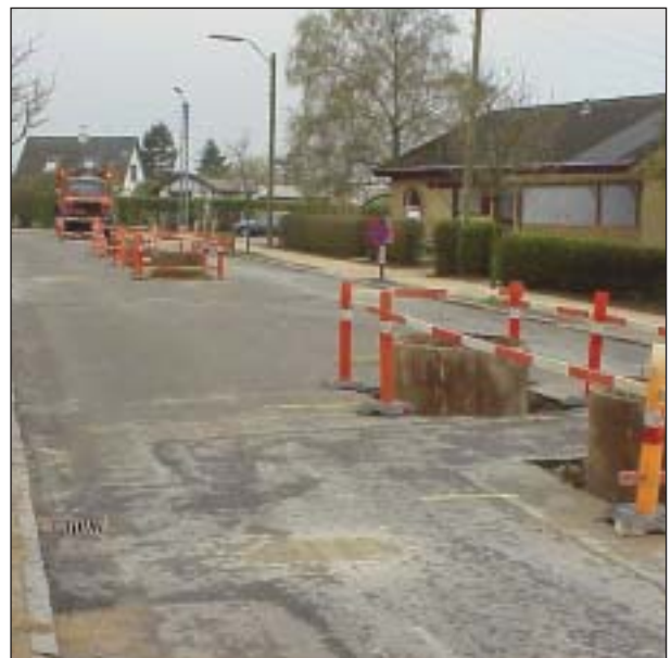
Vertical supports positioned above lateral connections.
