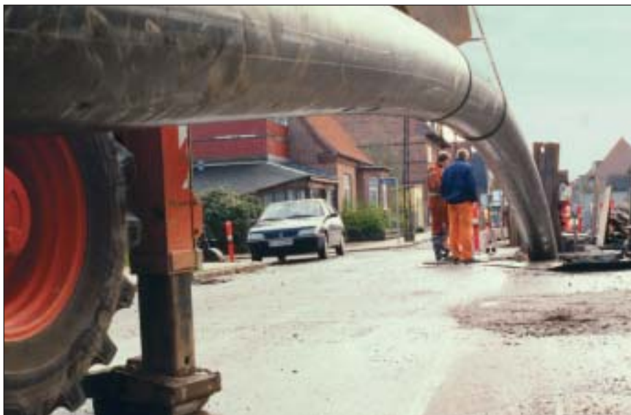
Sliplining work site.
