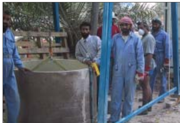
Mobile crane for lowering panels into a manhole.
