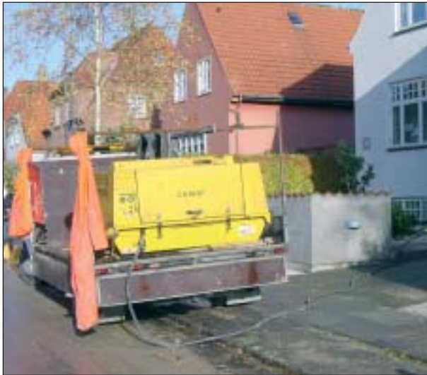
A typical example of impact moling from a basement.
