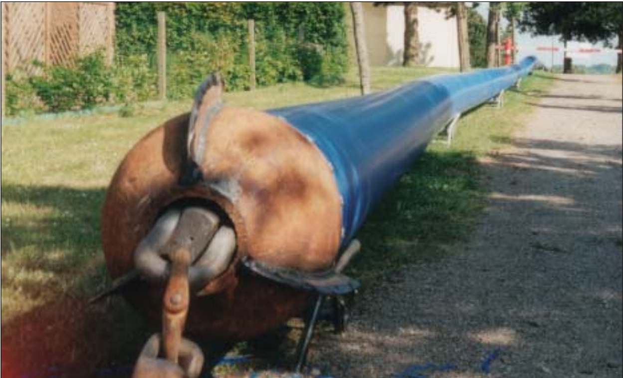
Fuse-joined PE pipe ready for installation.
