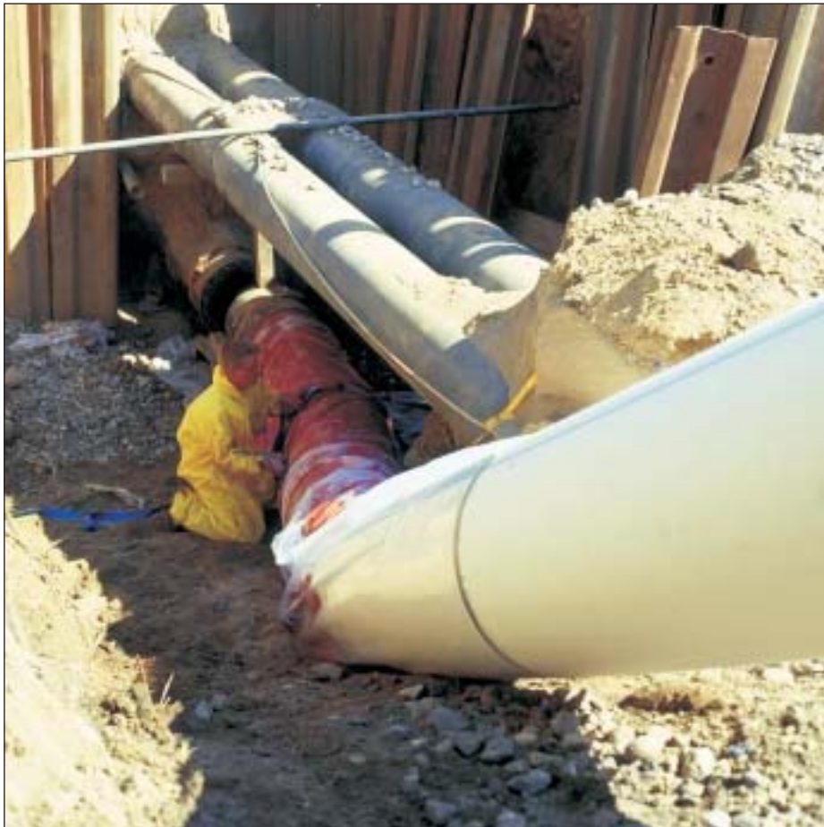
Installation under difficult conditions.
