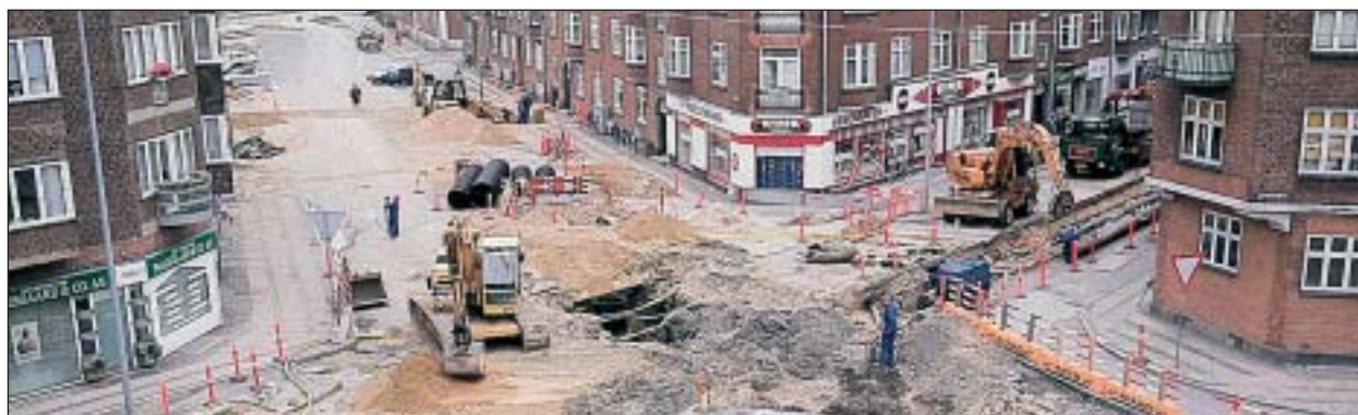
Space is required for open-cut work in city centres.
