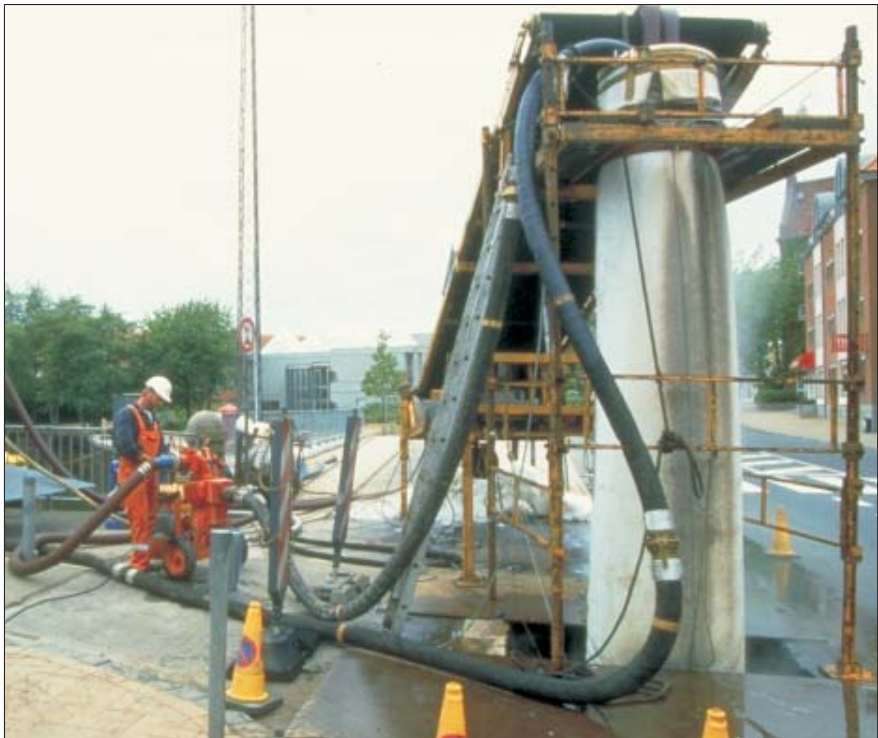
Cured-in-place lining
