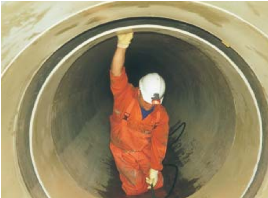
Fitting panels in an existing pipeline.
