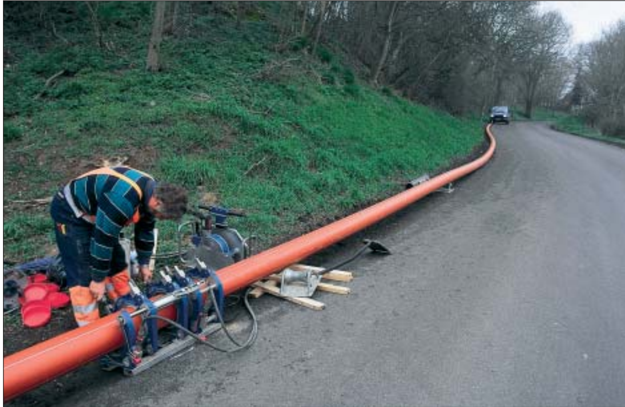
PE pipes are fusion-joined prior to installation.
