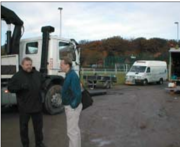
The control committee inspects work site layout.
