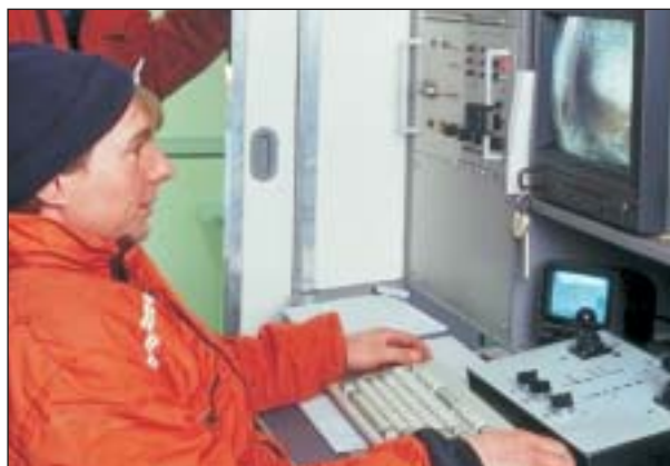
A CCTV operator inspects a lateral.
